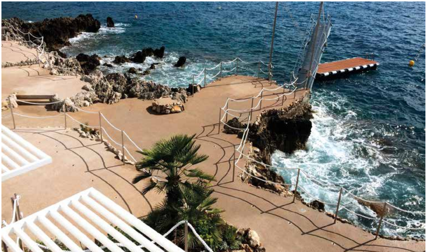
Vista Beach Palace, Roquebrune - Cap Ferrat ©MB Constructions
